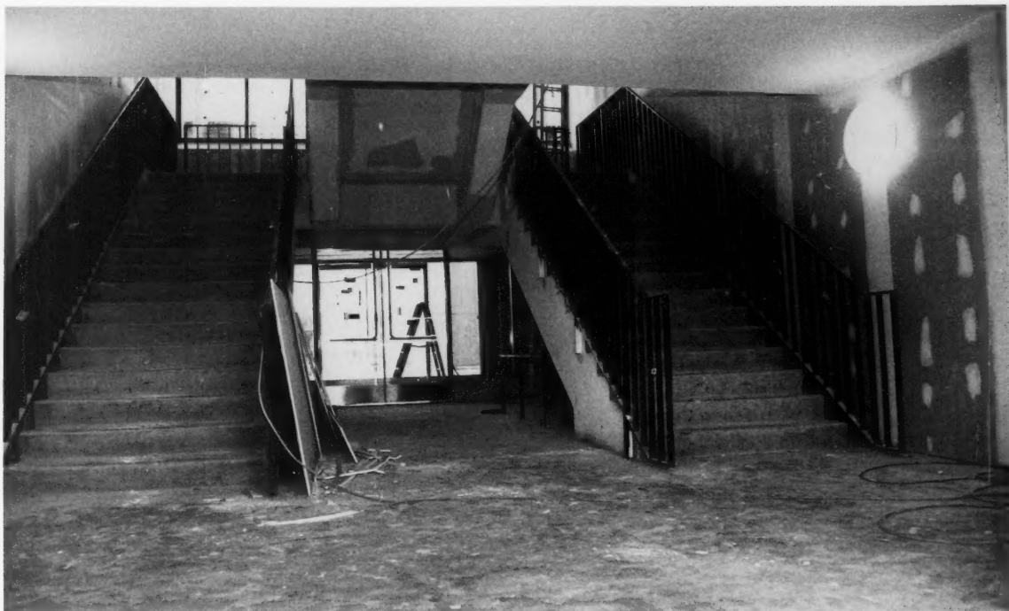
Design feature: a classroom building with double staircase.
